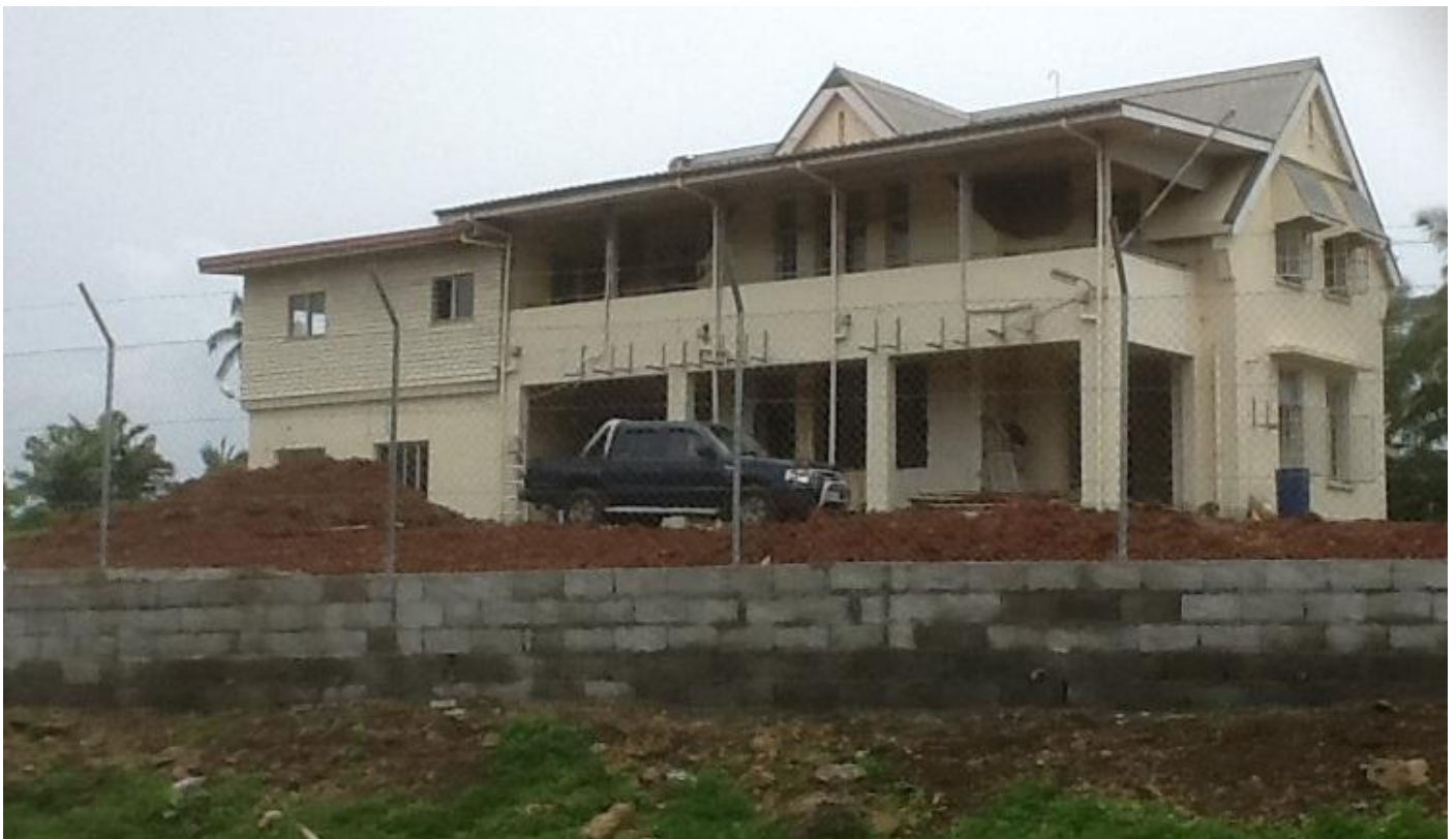
PIDF Secretariat at 56 Domain Road, Suva undergoing refurbishment
